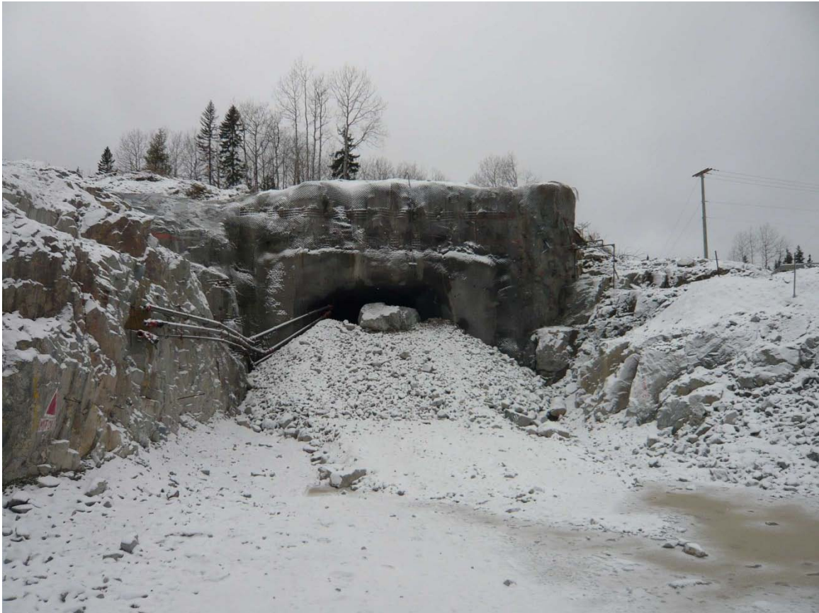
FIGURE 5-2 MAGUSI SITE – RAMP PORTAL – NOVEMBER 2008
