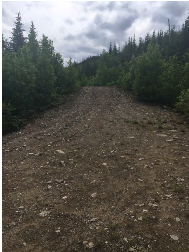
Photo 4: End of Access Road (to be upgraded) at Mine Site
