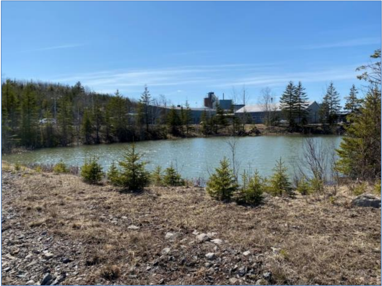
Figure 18-12: Storm Water Pond
