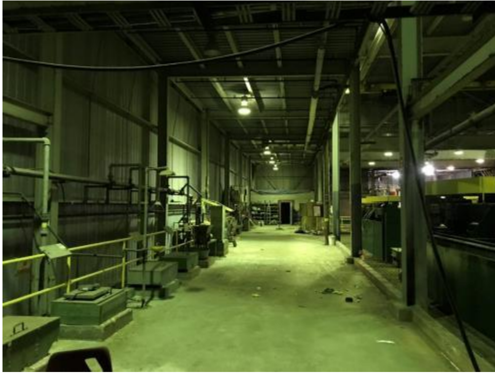
Figure 18-45: Large Main Deck Maintenance Bay
