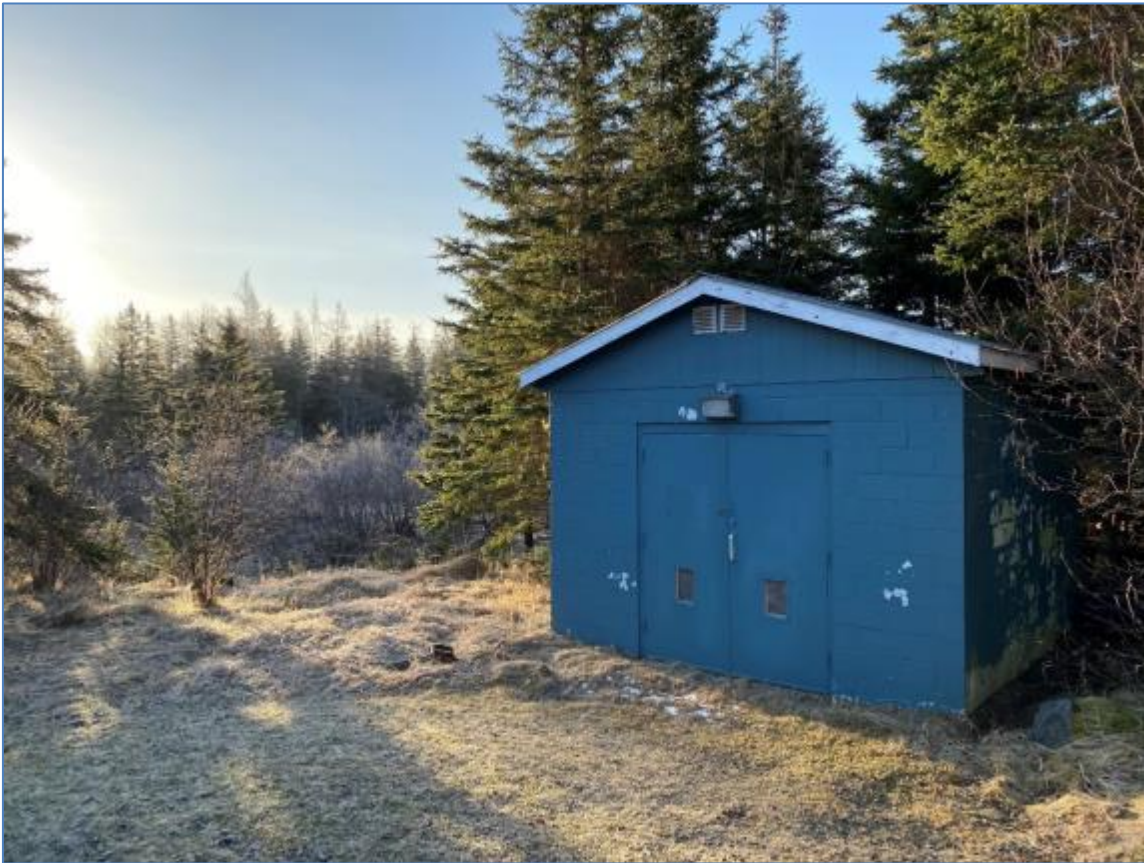
Figure 18-8: Pumping station at Gay's River
