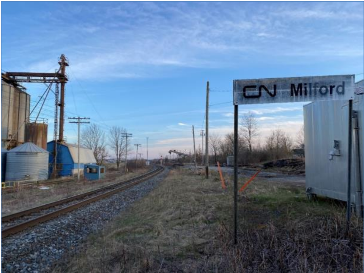
Figure 18-67: CN Milford Railway Siding
