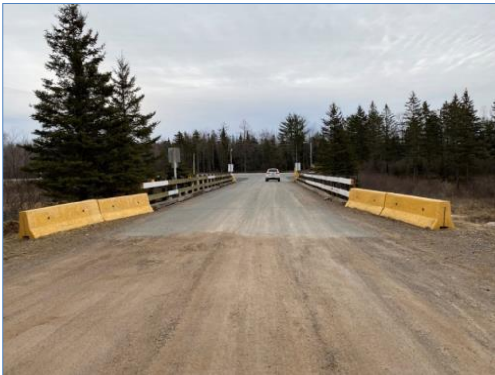
Figure 18-71: ScoZinc's Bridge & Highway Access
