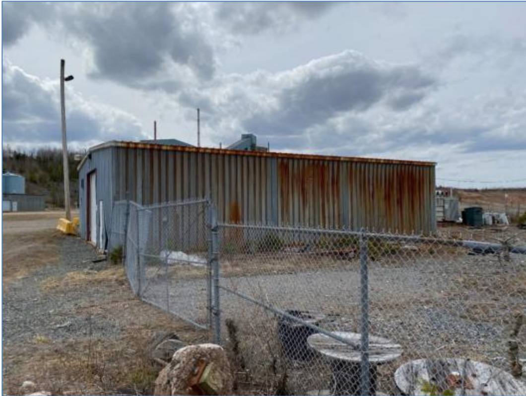
Figure 18-51: Cold Warehouse and Storage Yard
