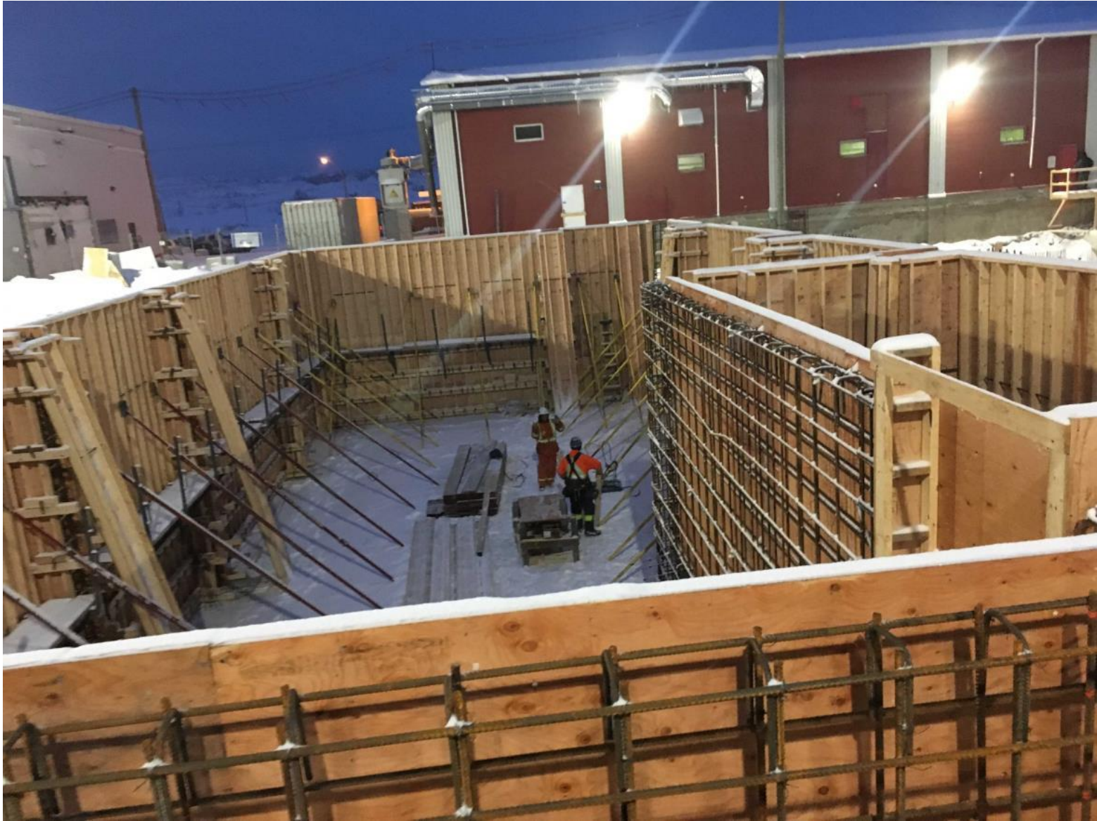
Picture 4: Hoist Building Construction: Main concrete slab pour
