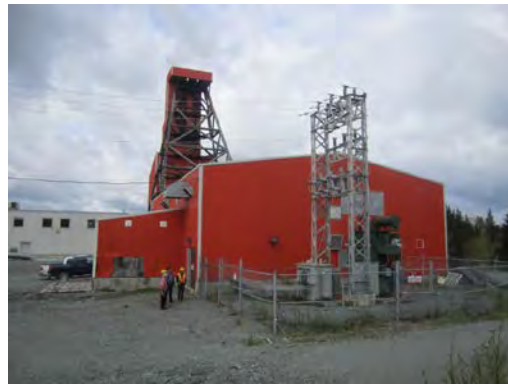
Hoist Room, #7 Headframe, Substation
