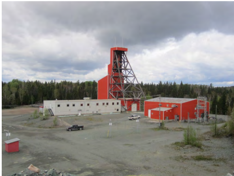
Office, #7 Headframe and Hoist Room
